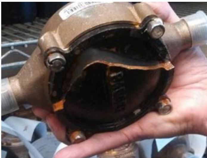
Broken Water Meter, Madison Water Utility: January 8, 2014
