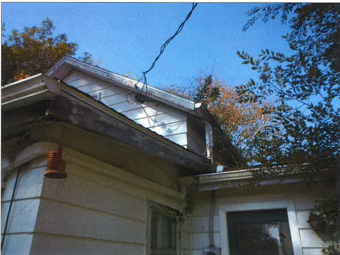
SOFFIT – FASCIA - GUTTERS
