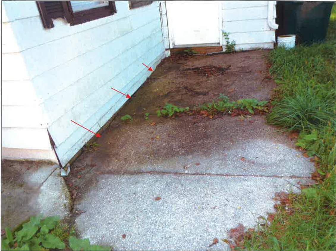
AREA OF SINKING CONCRETE (NORTH SIDE)
