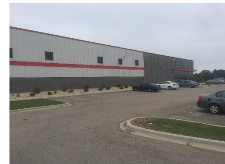
The above images, plus those included on Map 17, represent the Town's desired building quality in the Highway 12/18/N Interchange Area.
